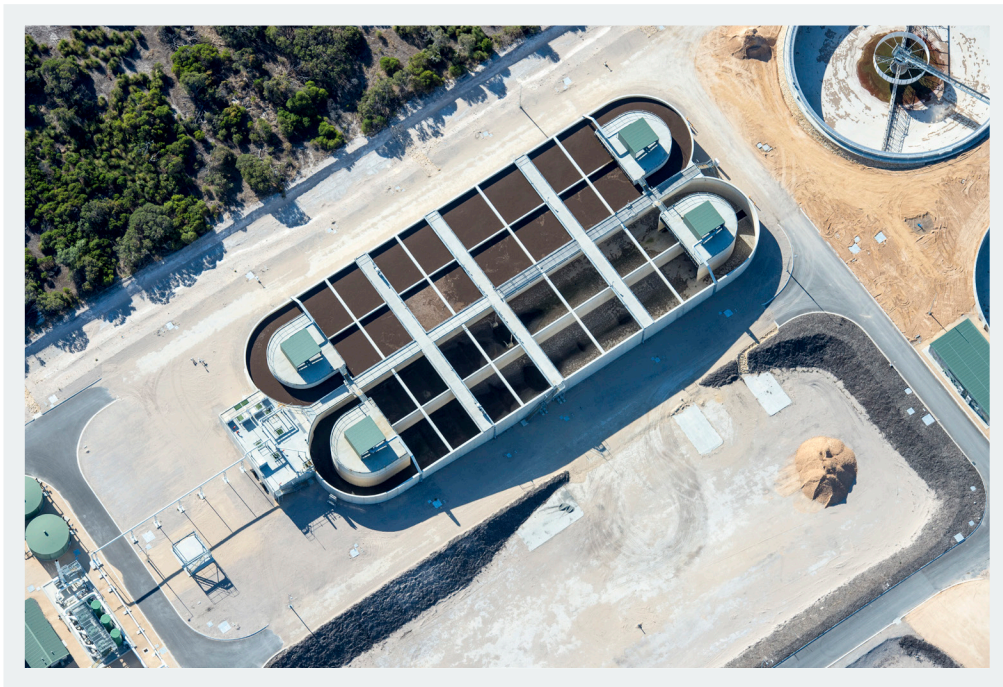
DBS Racetrack OXIDATION DITCH
